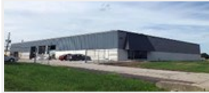
PARK FLETCHER BUILDING 4 2832 Rand Road Indianapolis, IN
