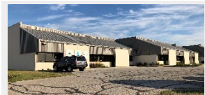
PARK FLETCHER BUILDING 15 2710 - 2762 Rand Road Indianapolis, IN
