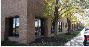
PARK 100 – BUILDING 79 7750 – 7796 Moller Road Indianapolis, IN
