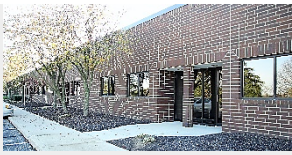
PARK 100 – BUILDING 109 5751 – 5827 W 73 rd Street Indianapolis, IN
