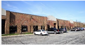
PARK 100 – BUILDING 80 7702 – 7742 Moller Road Indianapolis, IN
