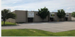
PARK 100 – BUILDING 31 8446 – 8450 Moller Road Indianapolis, IN
