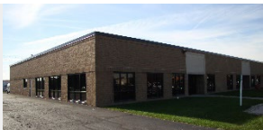
PARK 100 – BUILDING 112 5755 – 5855 W 74 th Street Indianapolis, IN
