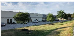
PARK FLETCHER BUILDING 27 2701 Fortune Circle East Drive Indianapolis, IN
