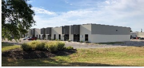
PARK FLETCHER BUILDING 16 5315 - 5365 W Minnesota Street Indianapolis, IN
