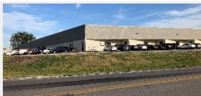
PARK FLETCHER BUILDING 22 1930 - 1944 Executive Drive / 5510 - 5522 Dividend Drive Indianapolis, IN
