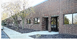
PARK 100 – BUILDING 109 5751 – 5827 W 73 rd Street Indianapolis, IN
